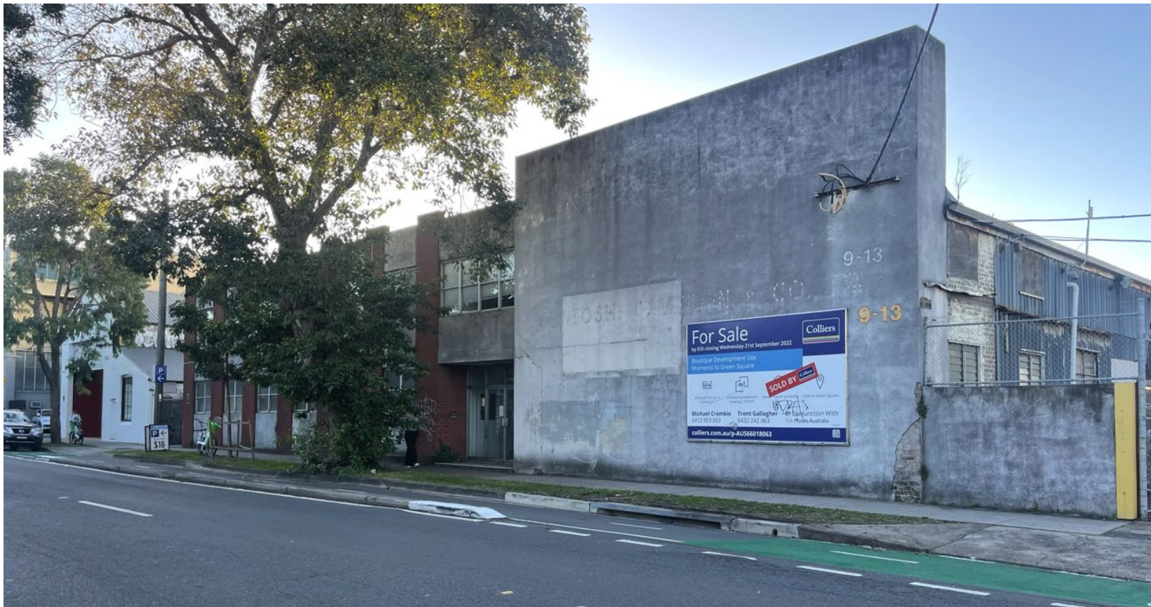
warehouse opposite the site at 9-13 Bourke Road
