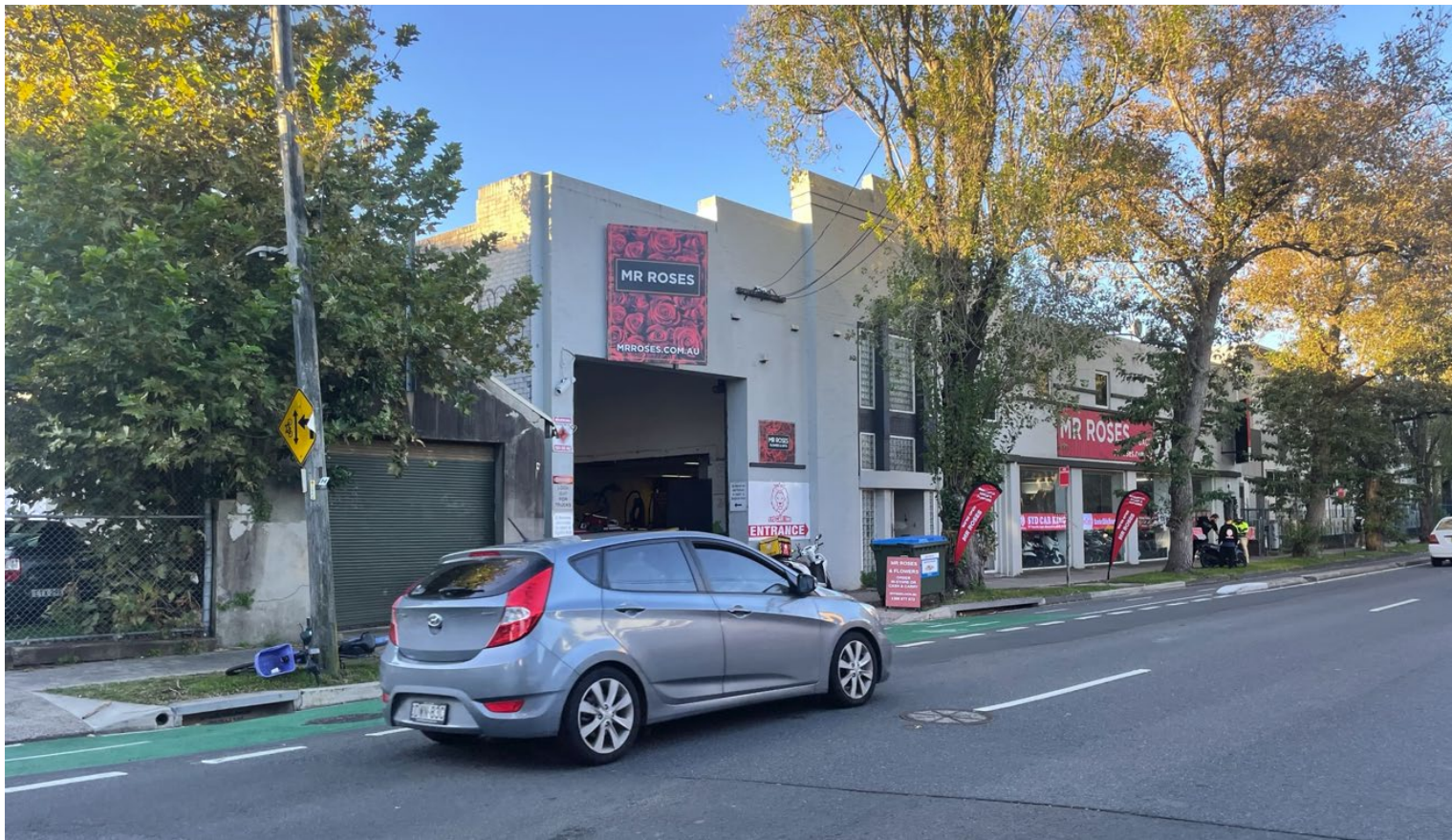
warehouse opposite the site at 5-7 Bourke Road
